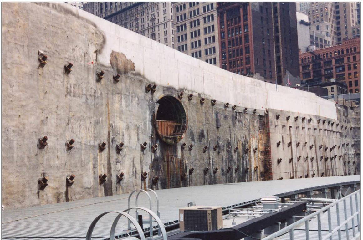
View showing remaining portion of the south tube, visible in the east slurry wall 4
