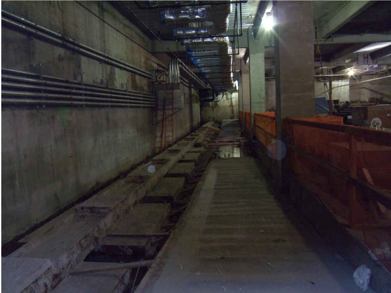
Photo of the box beam column from the north tower
