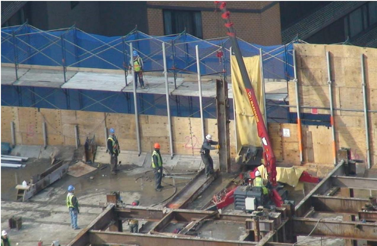
**Spyder Crane** – the small size and maneuverability of these mini-cranes allow them to be used where other cranes cannot go. On the 130 Liberty Street project the mini-cranes are used to access the interior of the building, hold steel in place, and lower steel onto the deck.
