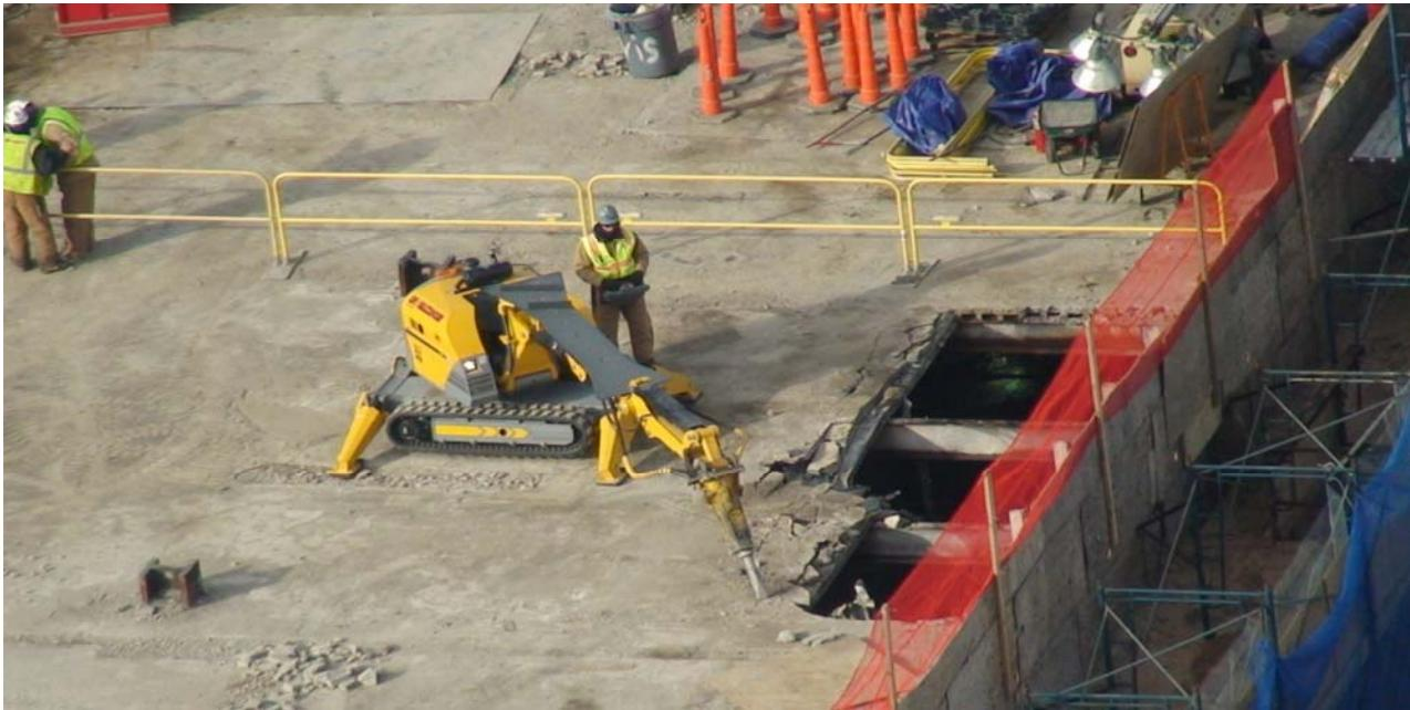
**Brokk Demo Robot** – used to break the concrete floor panels at 130 Liberty Street. The remote control access allows for construction workers to conduct the operation at a safe distance from demolition of the concrete flooring.
