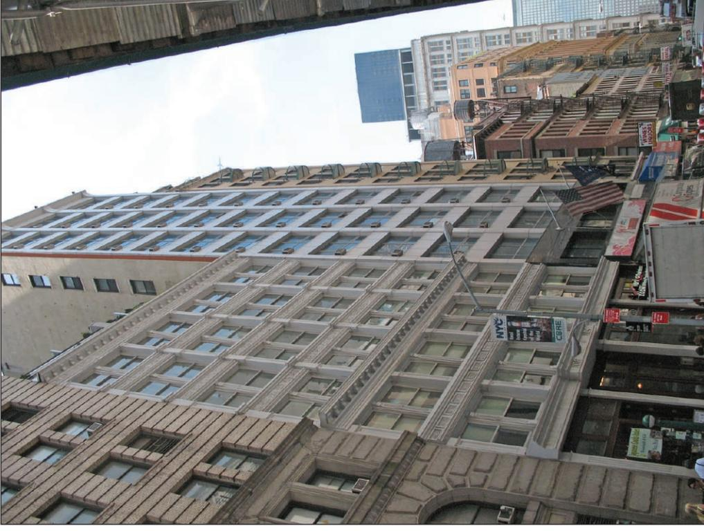
**4** The Fulton Chambers Building, (102-104 Fulton Street), the seven-story, eight-bay structure with cast-iron façade, pictured in the center of the photograph, was built ca. 1895
